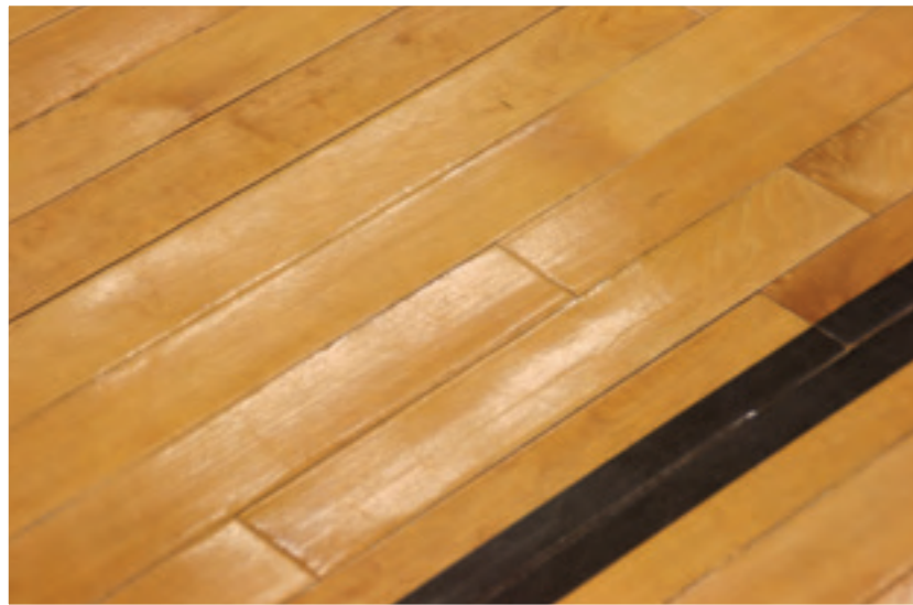
(Above) A plumbing-related failure released water down the gymnasium wall, and under the center of the affected half of the gym. This water loss was more highly concentrated and directional, causing a higher range of damage into a smaller area.
