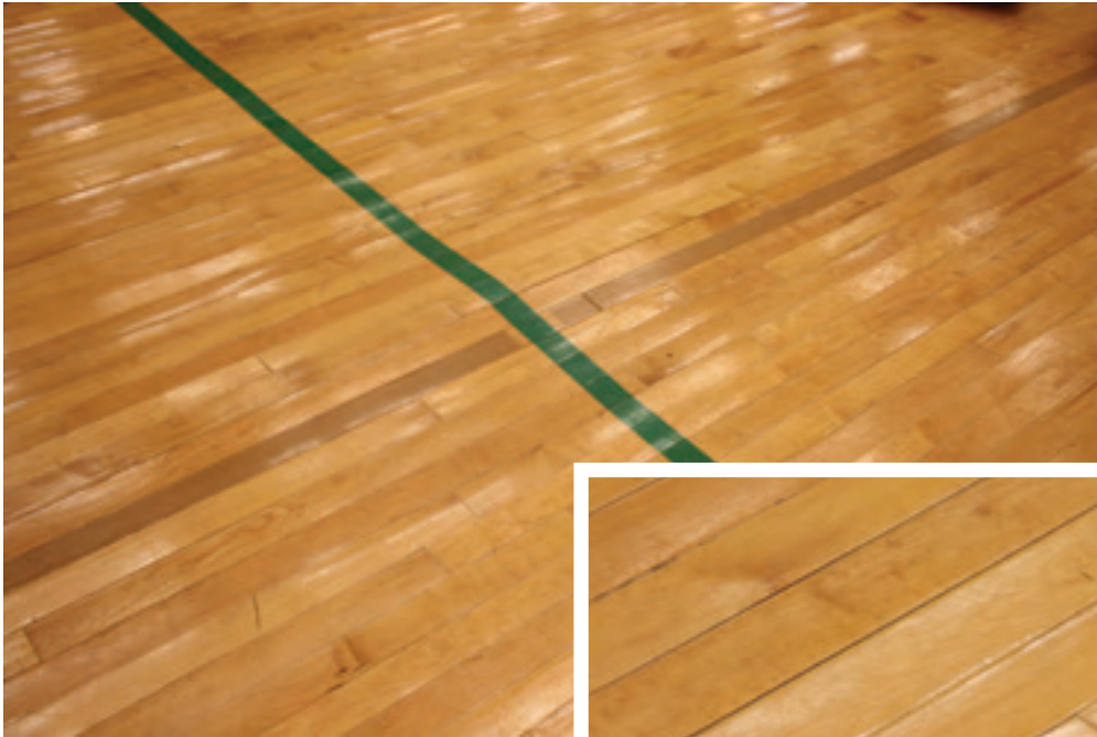
(Above) A plumbing-related failure released water down the gymnasium wall, and under the center of the affected half of the gym. This water loss was more highly concentrated and directional, causing a higher range of damage into a smaller area.
